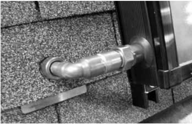
Figure 10 - Copper Flashing
