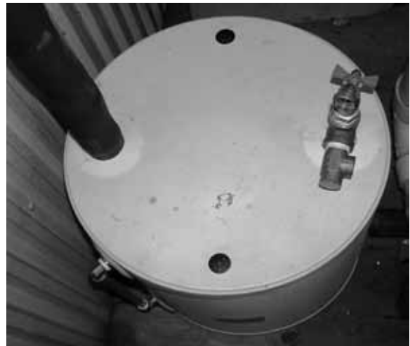
Figure 13 - Pressure Relief Valve
