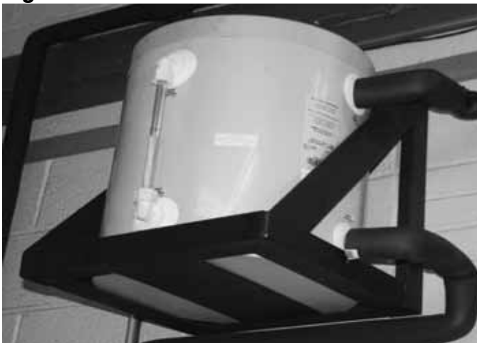
Figure 14 - Drainback Tank Relief Valve Piping
