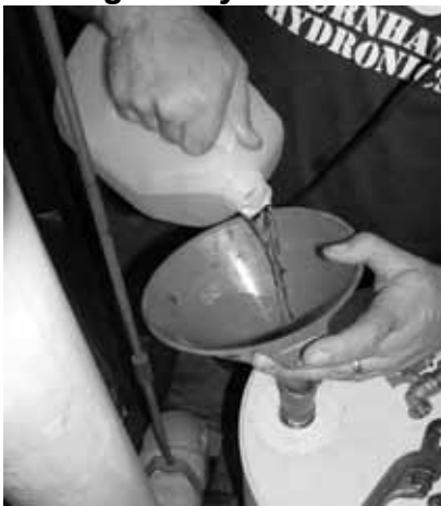
Figure 19 - Filling the System
