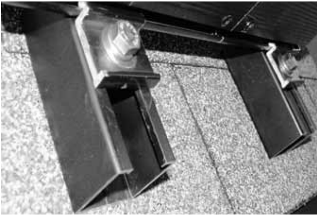
Figure 8a: Mounting Clips for Flush Mount
