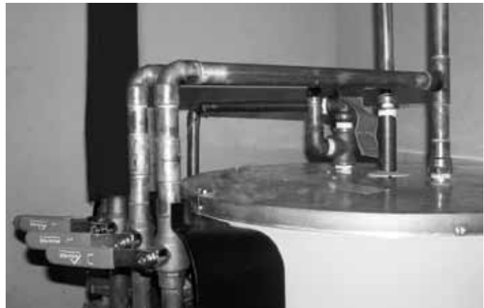
Installing the Differential Control
