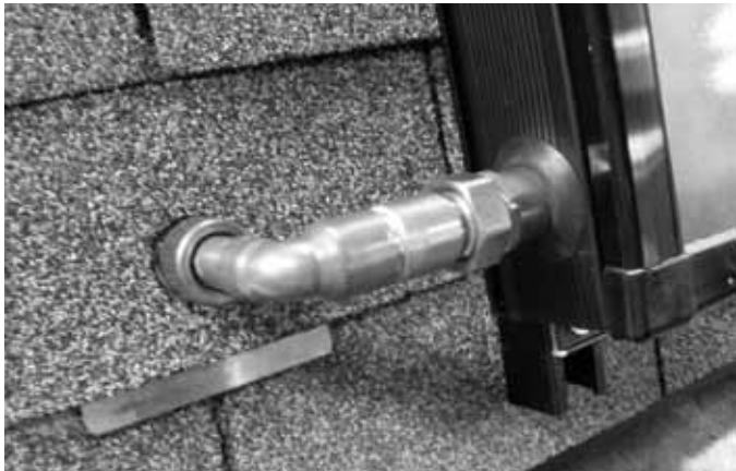
Figure 10 - Copper Flashing
