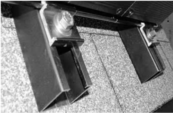
Figure 8a: Mounting Clips for Flush Mount
